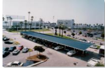
30kW PV Installation
